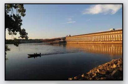
Featured in this year's report are photos of Wilson Dam. Construction of the dam began in 1918 and was completed in 1924. The dam is 137 feet high and stretches 4,541 feet across the Tennessee River. Wilson Dam is a hydroelectric facility with 21 generating units. Photography by L. Wray Dillard.
